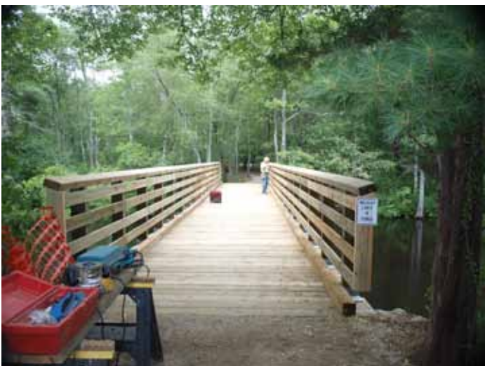
Pedestrian and Equestrian Bridge into Bradley Palmer State Park is now open for use after extensive work. See related story on page 8.
