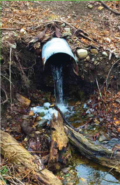
Before replacing culvert.
