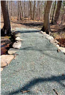
New culvert on the Lingerman Trail.
