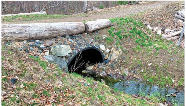
New culvert on Trail #23 in Willowdale.
